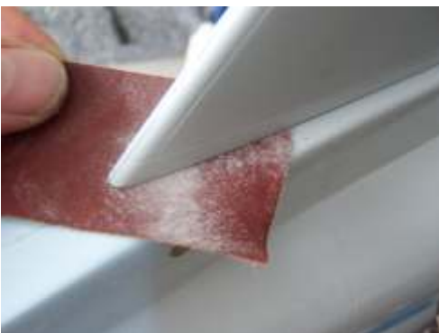
Check free movement, sand paper used for correcting disalignments
